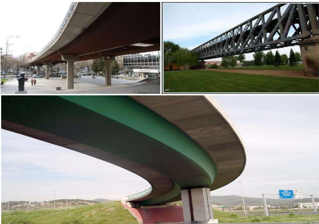
Image 3-12. Mixed structures with metal beams, lattice and box.
