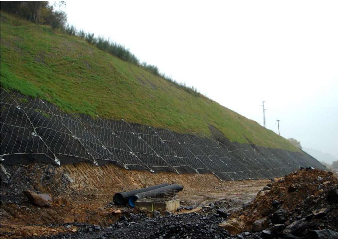
Image 3-27. Detail of geotechnical correction in slope.
