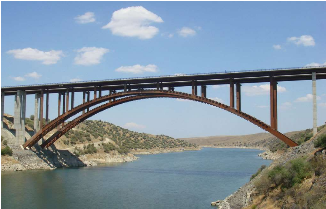
Image 3-18. Metal arch bridge.
