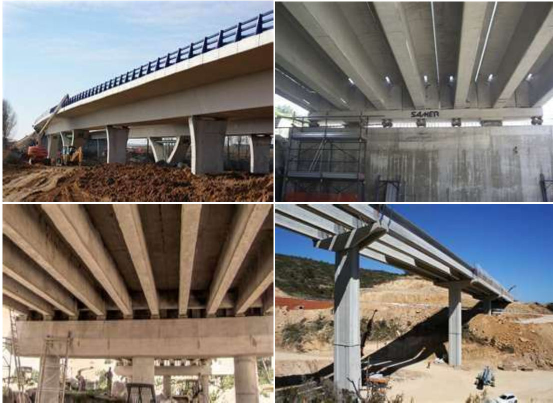
Image 3-9. Different types of prefabricated bridges with box girder beams or i-section beams.
