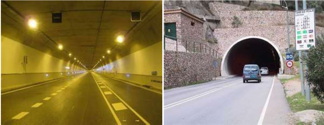
Image 3-21. Different images of tunnels with vault geometry.
