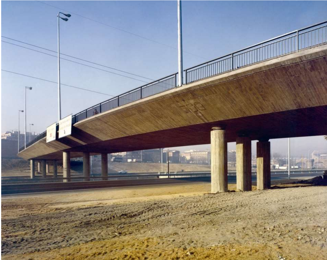
Image 3-14. Bridge post-tensioned on site with invariable edge.
