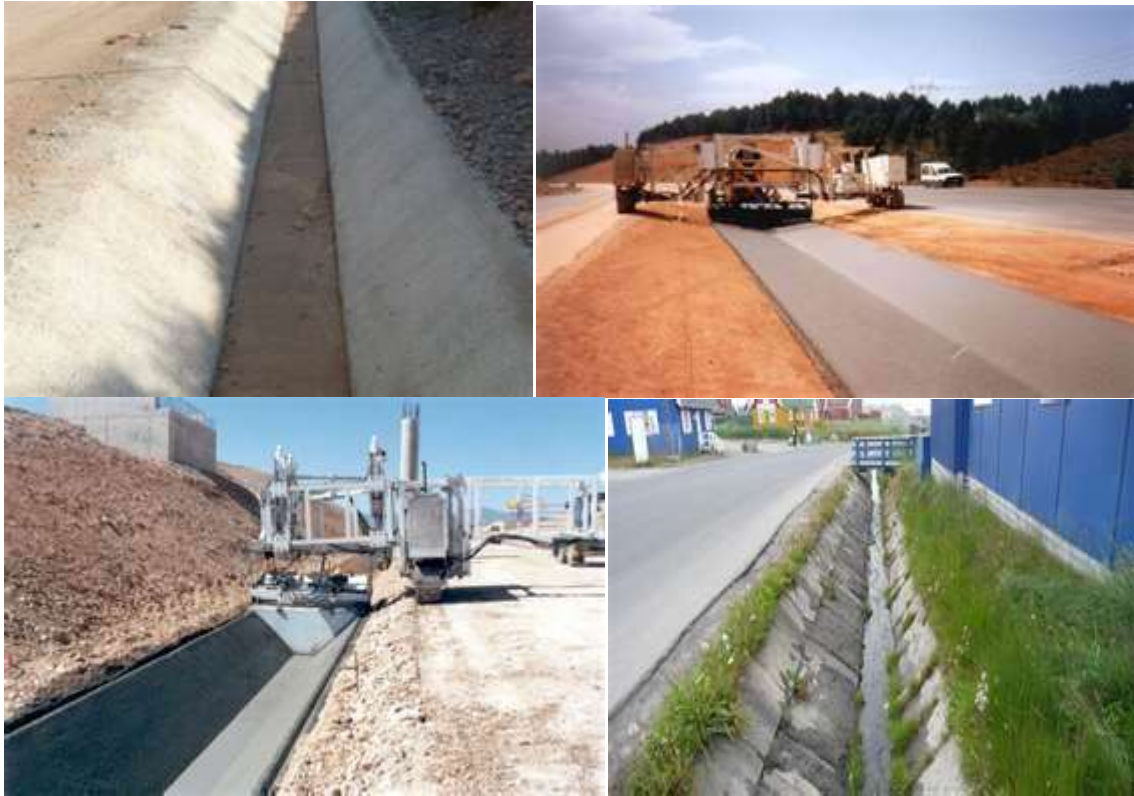
Image 3-6. Different types of ditches and their execution.
