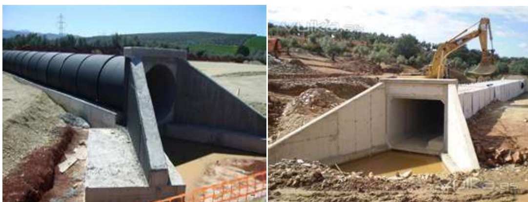
Image 3-23. Different images of transverse drainage works.
