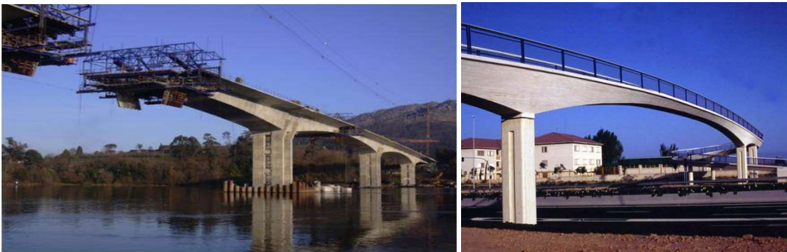
Image 3-15. Bridge post-tensioned on site with variable edge.
