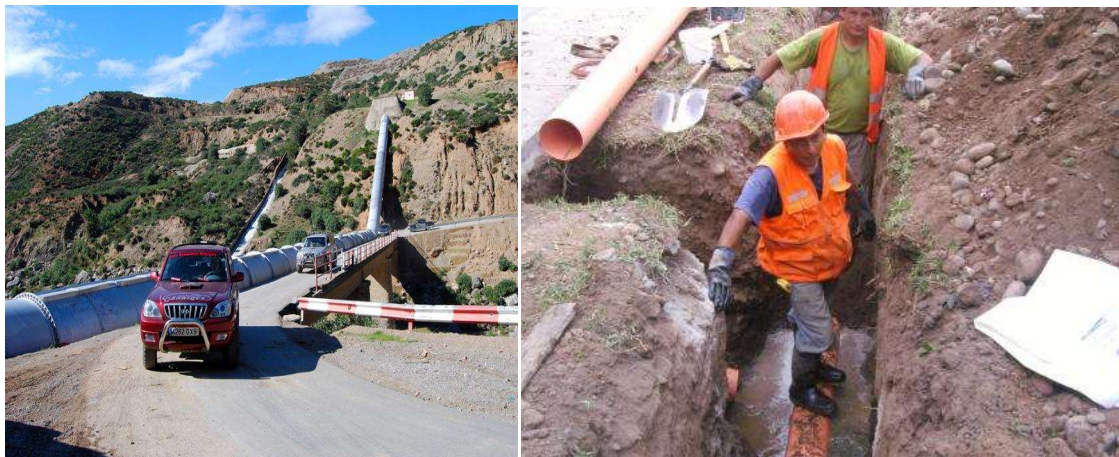
Image 3-26. Different images of replacement of services.
